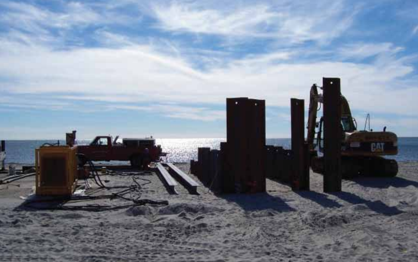
Creation of temporary cofferdam (sheet pile supported excavation) to bring submarine cable ashore.
