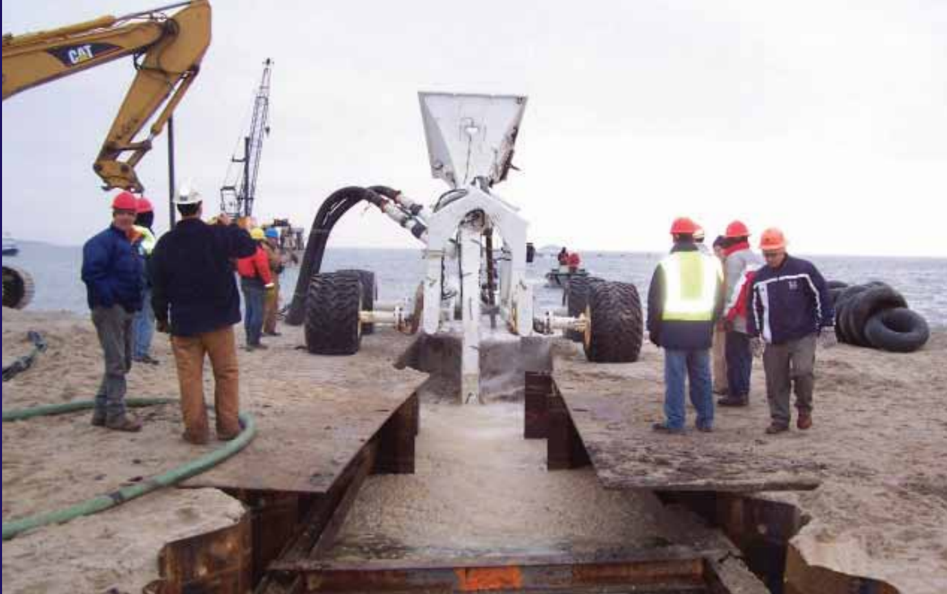
Submarine cable is fed through the plow, which will enter the water and travel along the seabed until making landfall on the opposite side of the water crossing.
